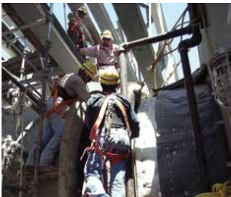
Fabric expansion joint installed over the manifold.
