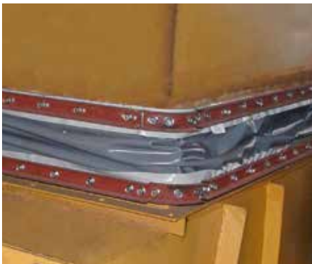
KE-Flex installed in an air duct.
